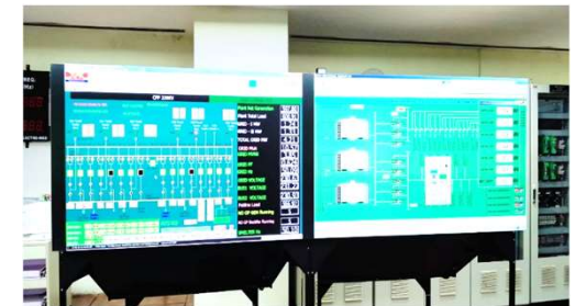
Installation of new BARCO make LVS
